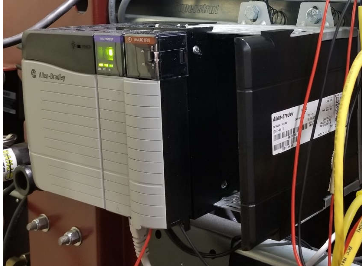
Figure 21. PLC with Ethernet/IP and Analog Modules.
